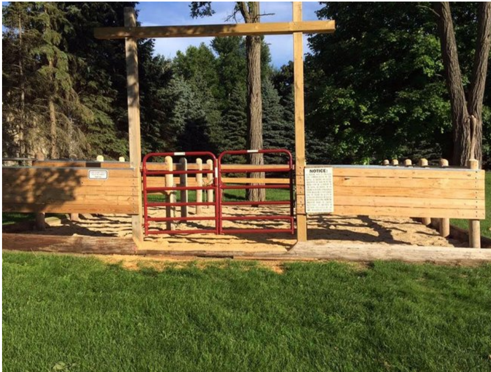
A corral for 10 horses was built in 2015 for the PFC Charles F. Duel Memorial Trailhead Park in Palmyra.
